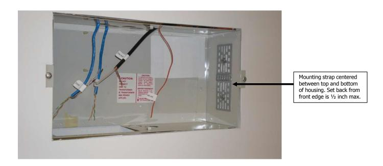
The view above shows the existing master housing with the right side strap installed. When mounting the left side strap, make sure the left and right straps are level. This will insure that the master is level when installed.
