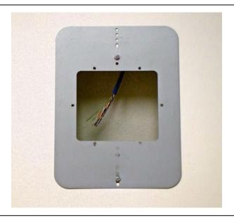
The view above shows the vertical adapter plate installed on the mounting ring.
