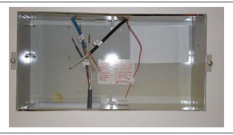
With the master removed, the housing should look something like this with all the wires disconnected and marked.
