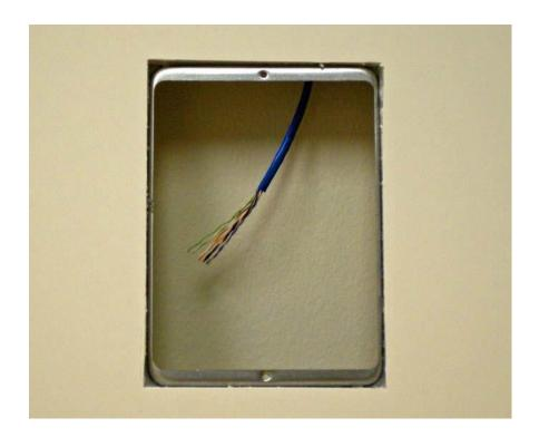
Once the old room station has been removed and the wires disconnected, the existing station hole with the existing rough-in should look something like the above picture.
