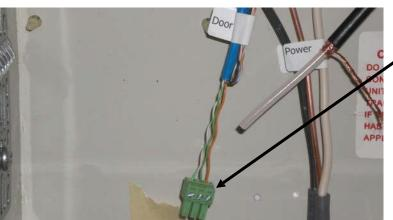
This view shows one of the green connectors attached to the existing wires.
